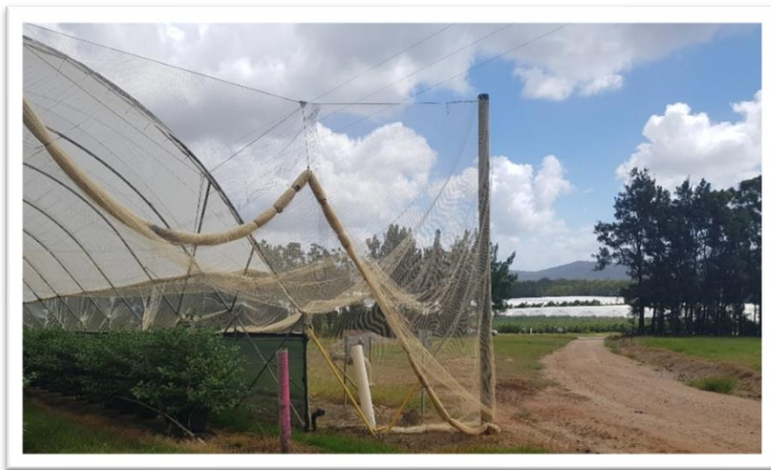
Costa, Netting over tunnel ends and sides.
